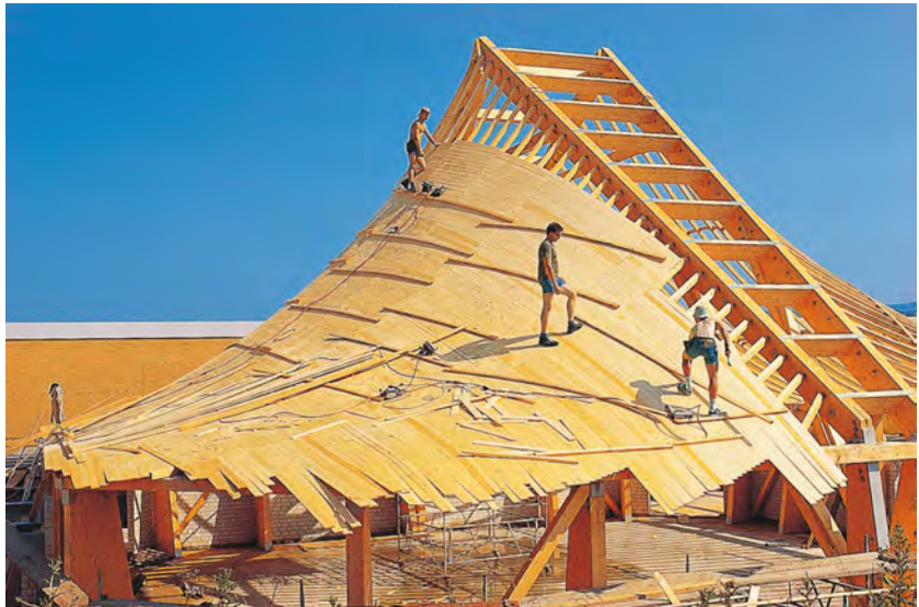
Fig. 3.30: The Wilkhahn production plant. Photos: Wilkhahn
