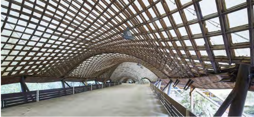
Fig. 3.32: The interior of the Mannheim Multihalle. Photo: Daniel Lukac
