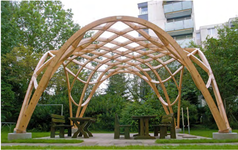
Fig. 5.10: The Z-Plus Pavilion by Création Holz, Blumer Lehmann AG, Design-to-Production GmbH, and SJB Kempter Fitze. Photo: Design-to-Production GmbH
