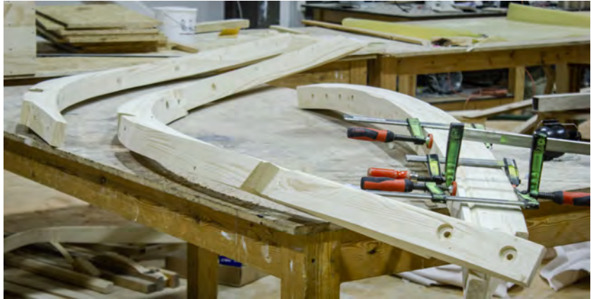
Fig. 6.57: Testing the assembly of individual components.
